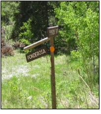
Figure 8. Combustible and non-reflective road signs.
