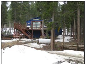
Figure 15. Home with combustible deck and open area under the deck.
